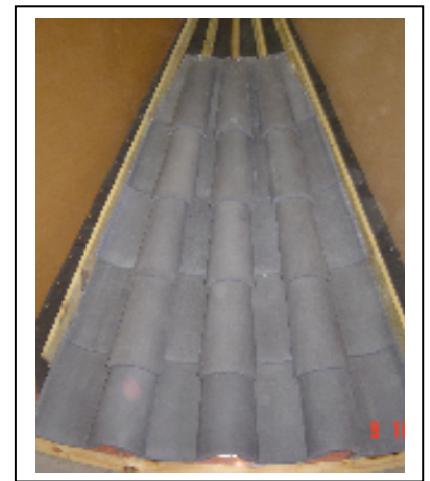
INSTALLATION OF COVERS
