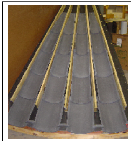
INSTALLATION OF PANS
